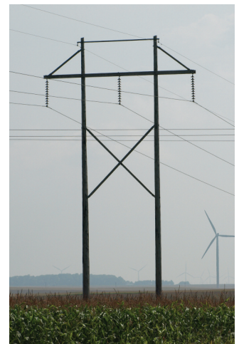
230-kV/345-kV H-frame transmission structure
