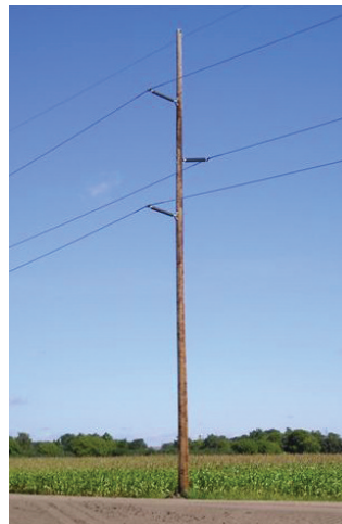
69-kV/115-kV transmission structure
