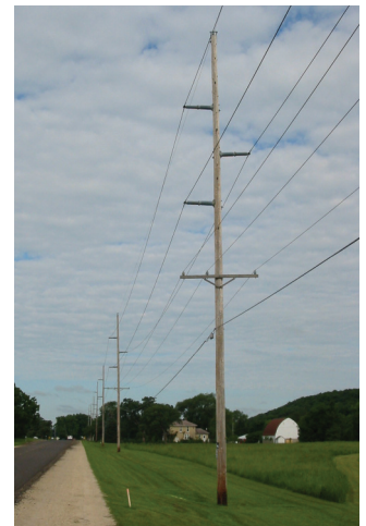
69-kV/115-kV transmission structure with distribution underbuild
