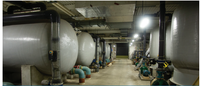
The Zoo's life support systems cycle water through pumps and tanks and filter out uneaten food, feathers and scales. Water is boiled and chilled to maintain an exact temperature and pH level, simulating an ocean environment.
