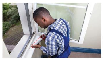
**2. SEAL AIR LEAKS WITH CAULK.** Applying caulk around windows, doors, electrical wiring and plumbing can save energy and money.
