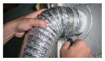
1. TRIM DRYER VENT. If your dryer vent hose is too long, your dryer is working harder than it has to, using more energy than necessary. The vent hose should be long enough for you to pull the dryer out a couple feet from the wall, but the shape of the hose should form a line — it should not have a lot of slack, with twists and curves. A shorter, unobstructed vent hose increases the efficiency of your dryer, dries clothing faster and reduces lint buildup, which can create potential fire hazards.
